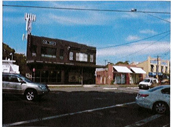
Plate 2-2 Commercial buildings at the southern portion of the site.
